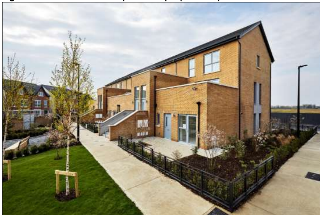
Figure 2.19 – Cairn Homes Duplex Example (Parkside)
